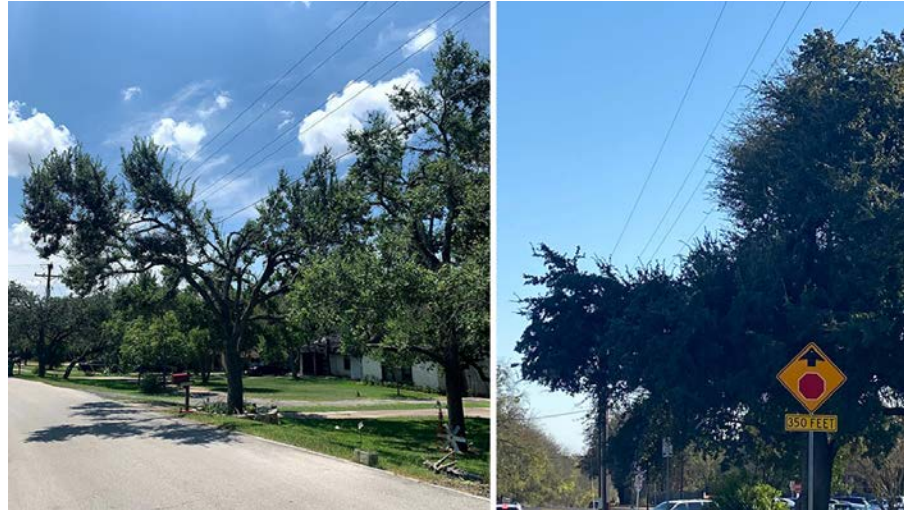
These examples of V-Cut (left) and L-Cut (right) directional pruning create challenges for accurate satellite-based encroachment detection.
